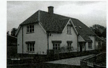
Home Field Black Window Cills / Pentic Boards / Chimney / Plain Tiles
