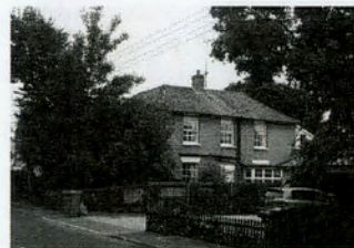
New Road All Bar Windows / Chimney
