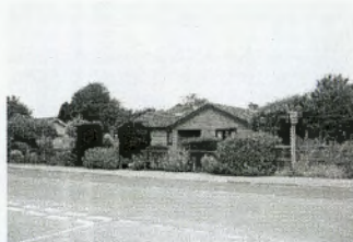
Station Road Black Fascias & Bargeboards
